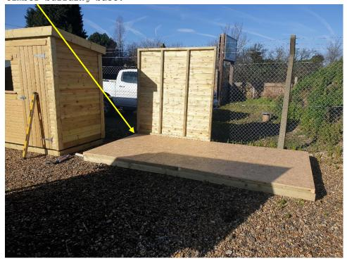
4.0- Fit the gable end panel and any additional side panels required-use the GP200 clear mastic on each joint, fix using  $3x\ 5x\ 70m$  screws- top middle and bottom of the panel joints.
