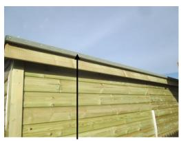
Proshop drip batten- roofing felt is nailed to the drip batten. The Proshop does not have side timber strips.
