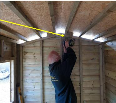
8.0- Ensure the walls are square to the floor and fix down using  $5 \times 70 \, \text{mm}$  screws- use 1x fixing to each upright timber spacing.
