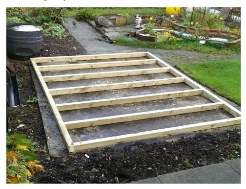
2.0- Lay out the timber building floor- check for level.
